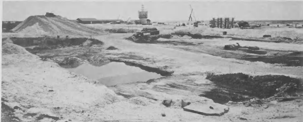
Foundations for several HDS units are rising, including the HDS process stack near the Vacuum Pipestill. Fundeshi pa varios unidad HDS ta lamtando, incluyendo un schoorsteen pa HDS cerca di Vacuum Pipestill.
